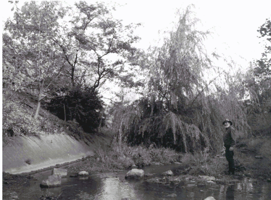
Figure 3.13. Riprap above and vegetation in the channel. Top : Looking upstream from the Tennessee Avenue Bridge. I-275 is at the top of the riprap-covered slope. Bottom : Looking downstream near the upper end of this channelized segment of the stream. Plants grow on most sediment in the channel. (Photographs by the author.)
