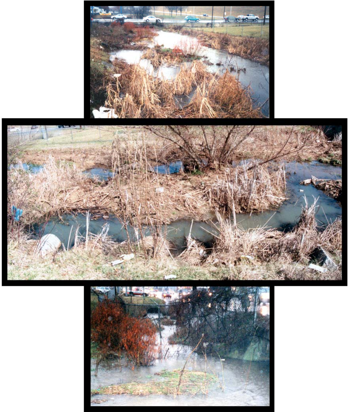
Figure 3.20. The area downstream from Merchant Drive. Top : Looking upstream towards Merchant Drive during a modest high water event. Middle : A "tributary" entering Second Creek from a 0.91 m diameter concrete pipe. Bottom : Looking upstream at storm runoff water running into Second Creek from a ditch along the southwest side of Merchant Drive. (Photographs by the author.)
