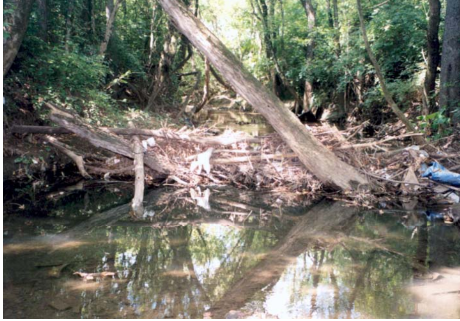
Figure 3.7. A woody debris dam between Bernard and Baxter Avenues. This view is looking upstream. (Photograph by the author.)
